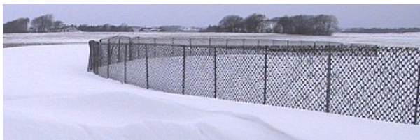
Figure 3: A snow fence placed on a field to stop blowing snow from moving father downwind.[expo-net.dk]
